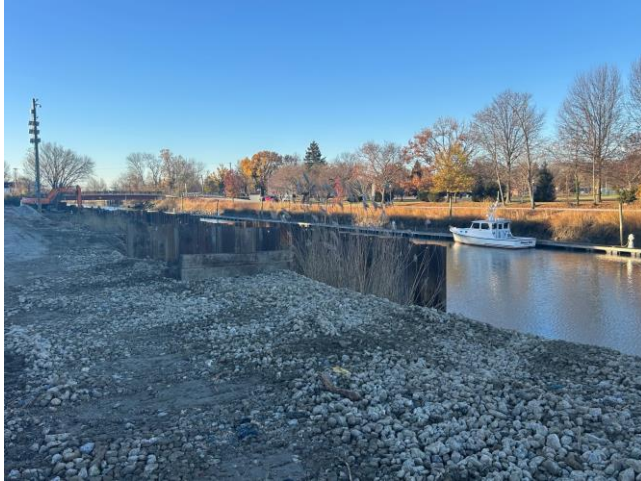
Coffer dam installation in first section with preliminary grading. (The view is looking northwest toward 5 th Street Bridge).
