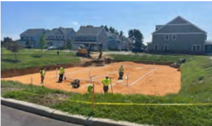
Bioretention Basin 3 – Early Stages
