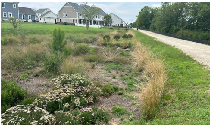
Bioretention Basin 1 – Fully Completed
