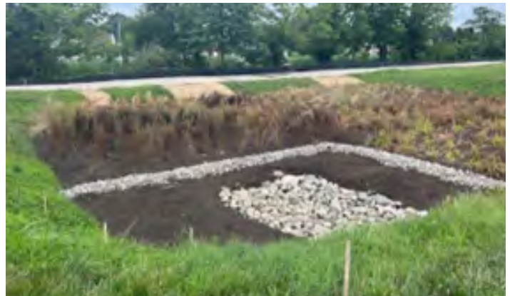
Bioretention Basin 2 – Partial Completion
