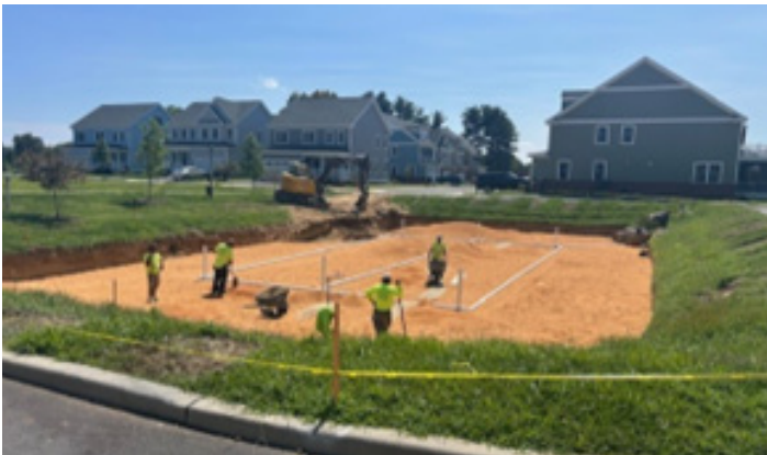
Bioretention Basin 3 – Early Stages
