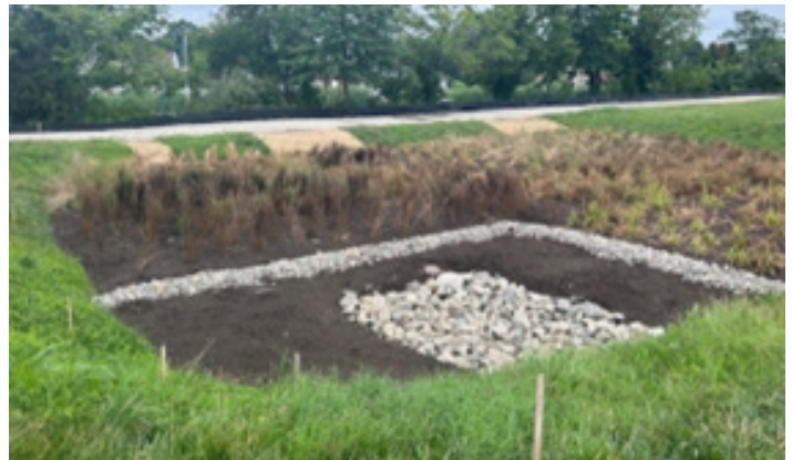
Bioretention Basin 2 – Partial Completion
