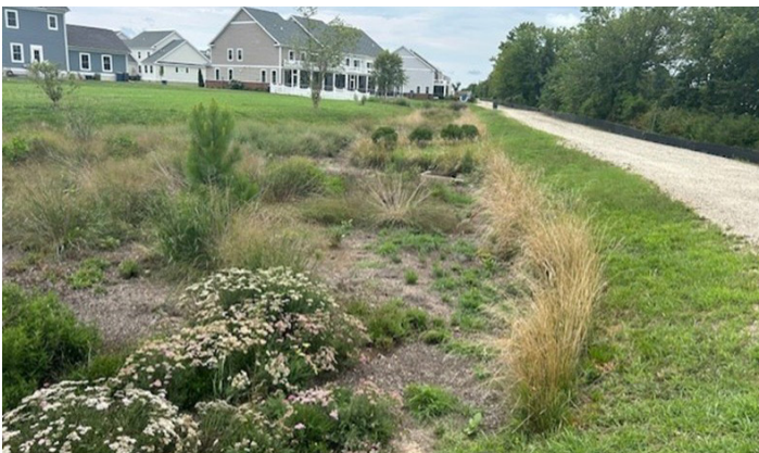
Bioretention Basin 1 – Fully Completed
