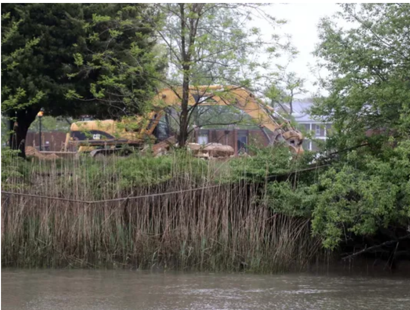
Construction along the Branch Canal that runs through Delaware City and the Fort DuPont property is shown on Monday. The site is being redeveloped into house and other buildings. (Photo: JENNIFER CORBETT/THE NEWS JOURNAL)
